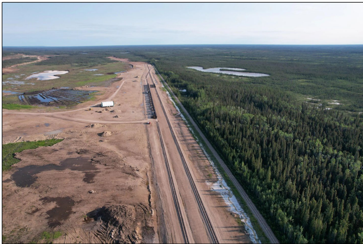
AWP Industries new rail-trucking trans-shipping facility, Enterprise, NT. See AWP Website .
